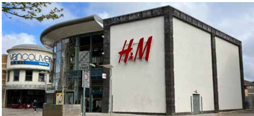
Existing H&M wall
