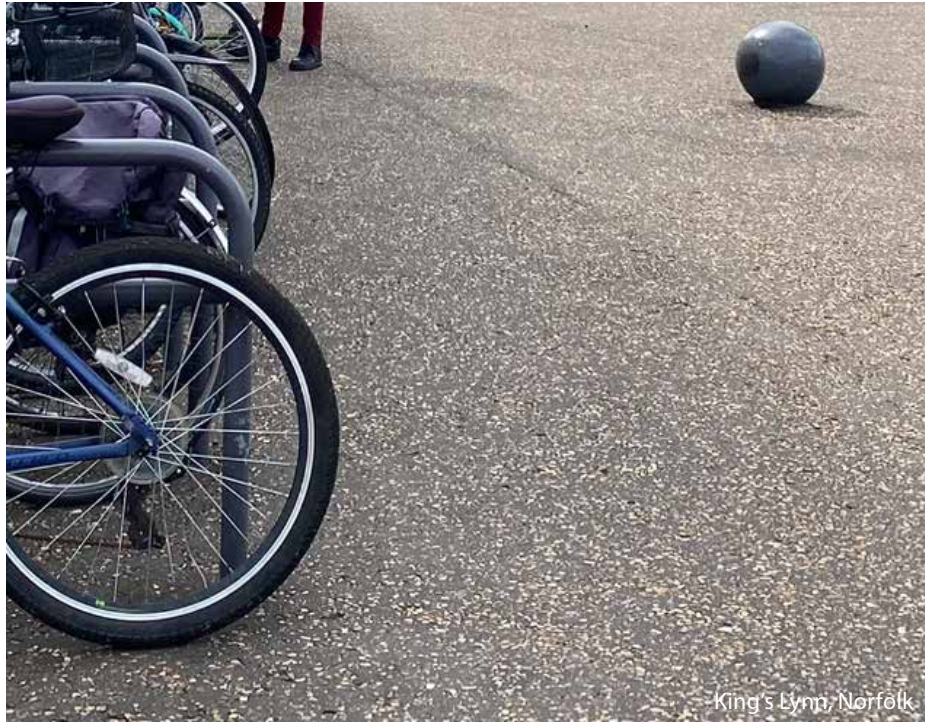
Asphalt surfacing with golden gravel
