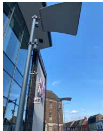
Vancouver Quarter lighting 4m light pole
