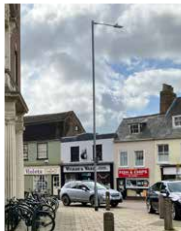
Blackfriars Street lighting 12m light pole
